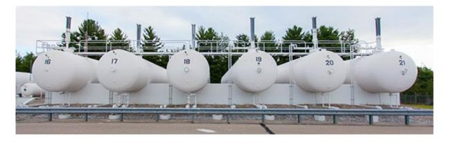
In addition to the cylinder sizes shown in Figure 15, commercial and business customers who consume large quantities of LPG use bulk storage tanks which come in various sizes for different applications. Bullet tanks can be used for commercial, industrial, and agricultural applications.
